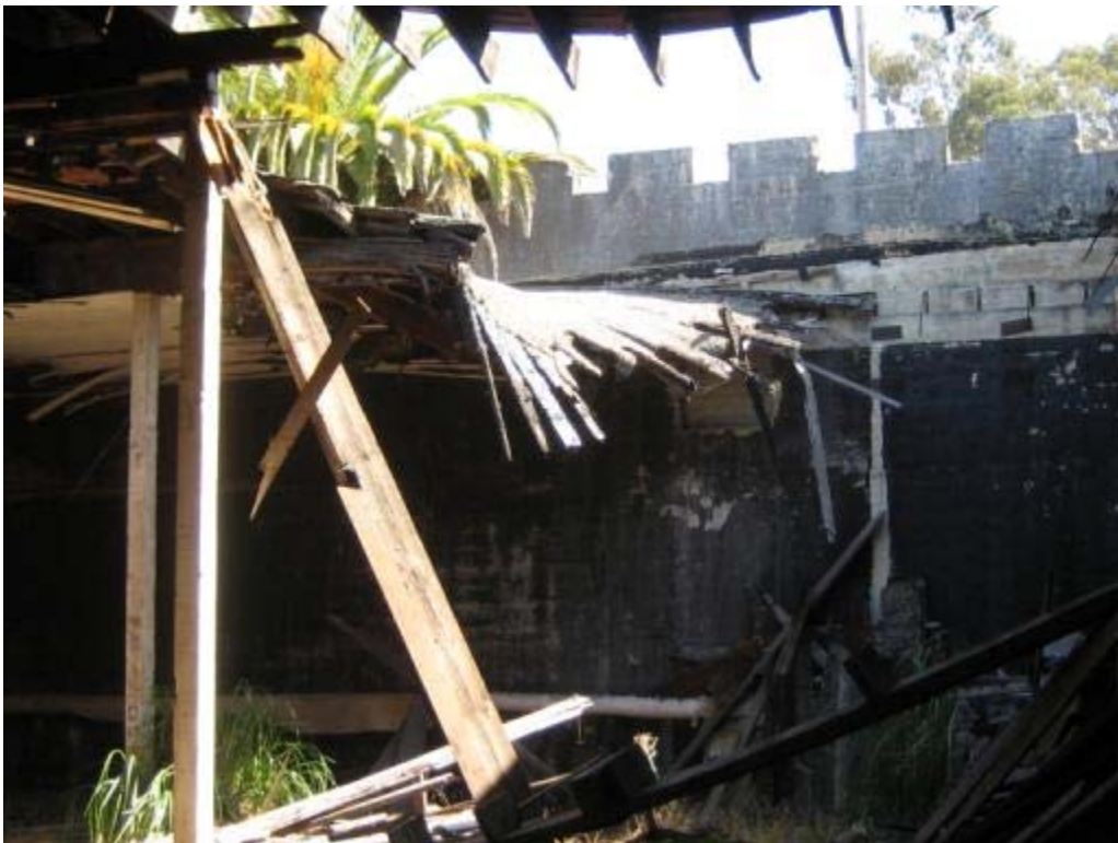
Lower portion of southern one-story area of Building 6. Note light coming through roof sheathing indicating membrane has failed.
